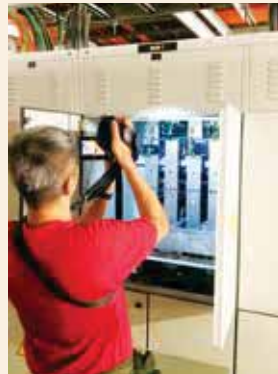
Figure 19: Thermography scanning of all the electrical panels at the building
