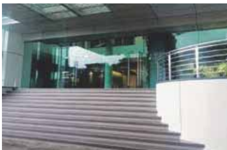
Figure 29: Upgrade staircase with anti-slip tiles
