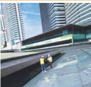
Figure 31: Upgrade of roof rainwater drainage system
