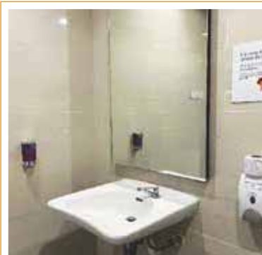
Figure 32: Upgrade of washroom in buildings
