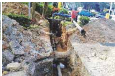
Figure 30: Replacement of underground domestic piping
